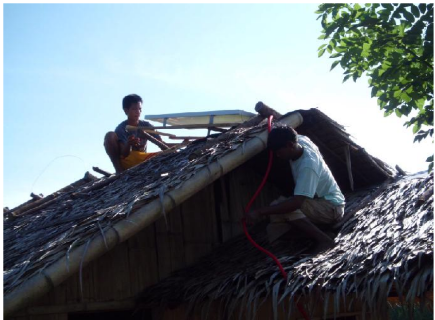
Installation of one of the ten solar generators for providing light the houses in the mountains.
